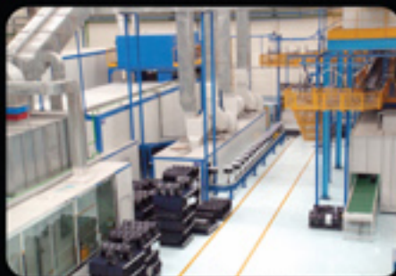
Dust free paint booth for high quality finishing
